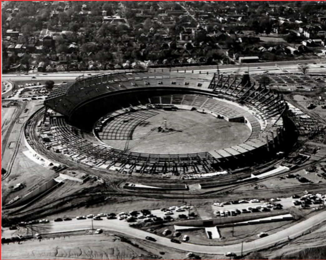
Aerial view of the Atlanta Stadium during its construction early in 1965
